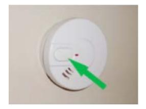
This is an example of a 9 volt battery operated smoke alarm. It only has one source of power and will be phased out of rental properties over the next 3 years.
