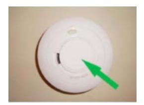
The below provides an example of a typical 10 year Lithium non-removable battery smoke alarm. These alarms are most commonly fitted to rental properties as there is no need for battery replacement.
