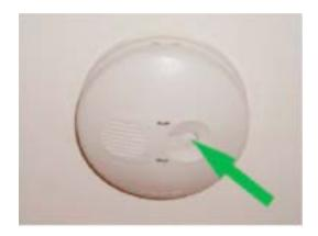
This is a common example of 240 volt mains powered smoke alarm with 9 a volt battery backup. It uses electricity from the light circuit in your home and in the event of a power failure will utilise the 9 volt replaceable battery installed.
